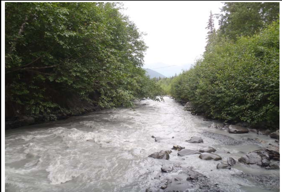
Bridge No. 0607 Br. Name Victor Creek Date 08/09/17 Inspector Murray / Murph Frame 4 Looking DS
