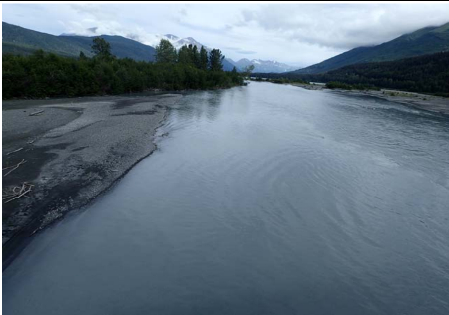
Bridge No. 0605 Br. Name Snow River Cntr Channel Date 08/09/17 Inspector Murray / Murph Frame 7 Looking DS 1
