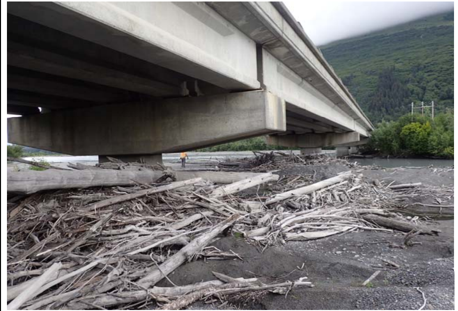
Bridge No. 0605 Br. Name Snow River Cntr Channel Date 08/09/17 Inspector Murray / Murph Frame 38 NE piers 2, 3, 4
