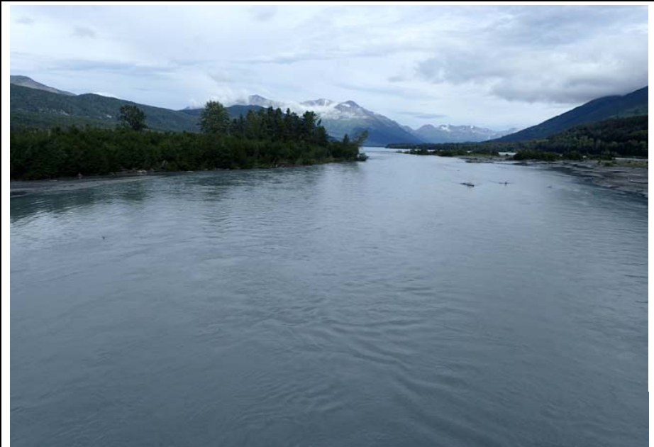
Bridge No. 0605 Br. Name Snow River Cntr Channel Date 08/09/17 Inspector Murray / Murph Frame 8 Looking DS 2
