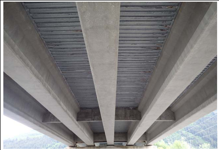
Bridge No. 0605 Br. Name Snow River Cntr Channel Date 08/09/17 Inspector Murray / Murph Frame 36 NE underside, typ.
