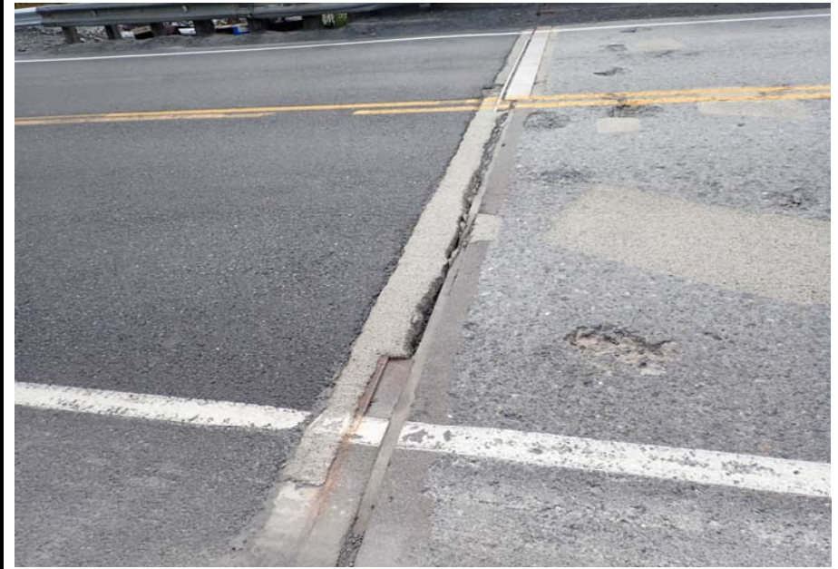
Bridge No. 0605 Br. Name Snow River Cntr Channel Date 08/09/17 Inspector Murray / Murph Frame 26 DS FE expansion joint
