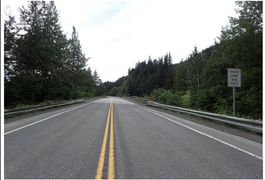
Bridge No. 0603 Br. Name Snow River West Channel Date 08/09/17 Inspector Murray / Murph Frame 2 Back at bridge
