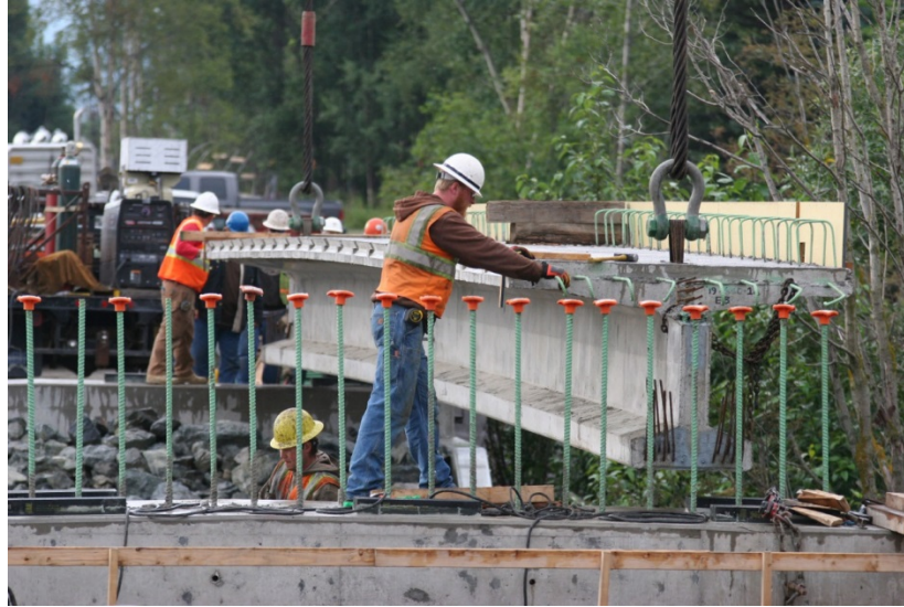
Figure 3 "Alaska-Style" Prestressed Girder Installation
