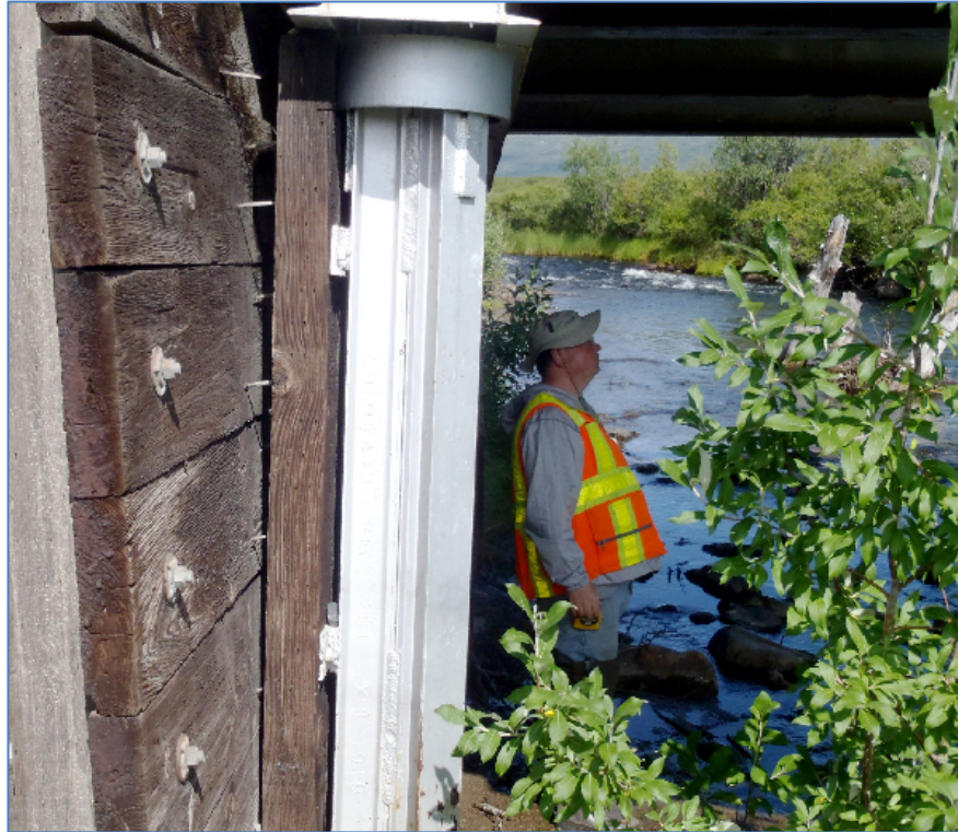
Figure 3. Rock Creek Backwall and Typical Rail Pile
