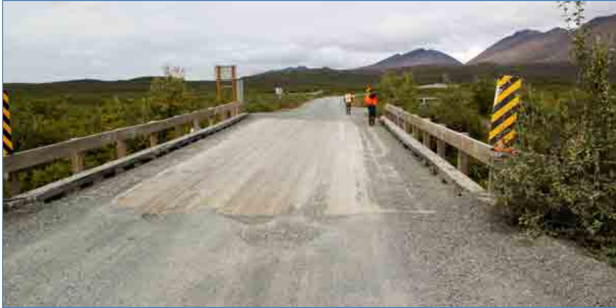
Figure 2. Rock Creek Bridge
