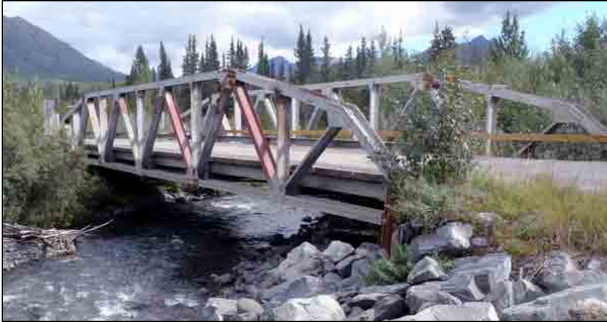
Figure 5. Chokosna River Bridge
