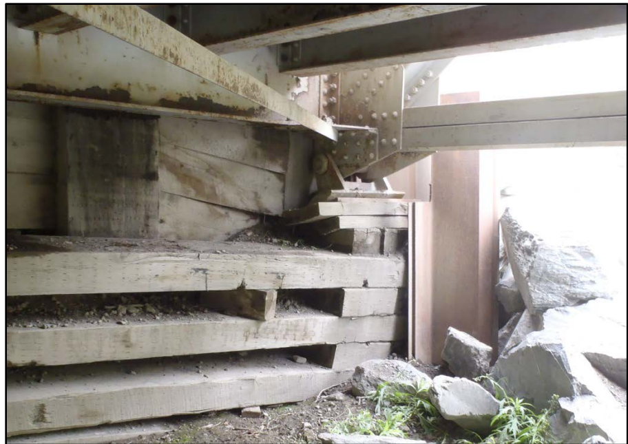
Figure 4. Chokosna River Bridge Foundation
