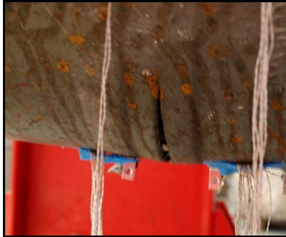
Figure 3-119: Second steel pipe rupture, Ductility 6, \Delta=9.67 in
