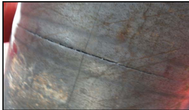
Figure 3-160: Crack opening on the pile leading to the first push of ductility 5, \Delta=9.1 in
