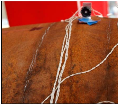
Figure 3-62: Tension cracking during the third pull, at 11 inches displacement, approaching the 13 inch displacement at ductility 4
