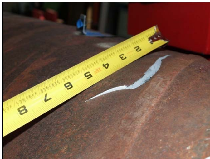
Figure 3-24: First rupture at the second pull of ductility 5 and a displacement of 17.07 inches
