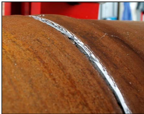
Figure 3-63: Rupture on top of the pile, ductility 4 pull 3, \Delta = 13 inches
