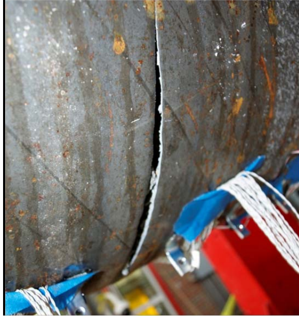
Figure 3-117: Steel pipe rupture, \Delta=8.40 in
