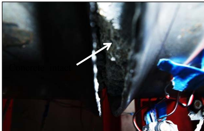
Figure 3-98: Rupture on underside of pile, Ductility 6, \Delta = 11.4 in
