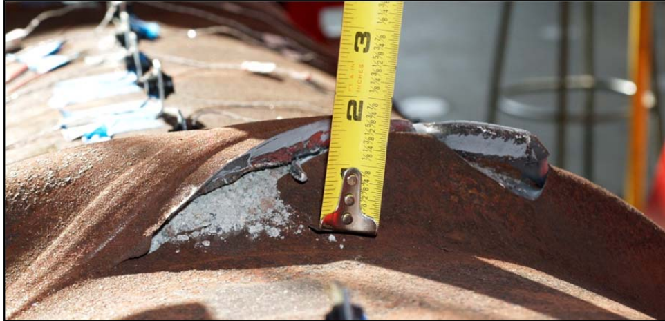
Figure 3-25: Rupture at the third push of ductility 5, a displacement of 17.07 inches
