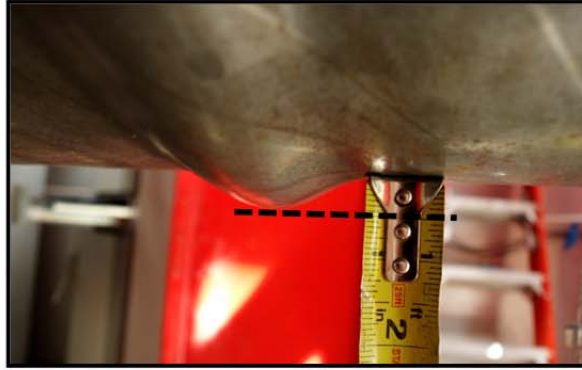
Figure 3-111: Buckle located under loading point, Ductility 3-3rd pull, \Delta=5.0 in
