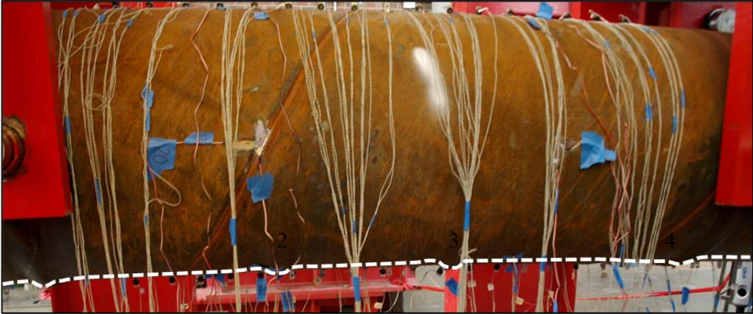
Figure 3-37: Four buckles located in the constant moment region at ductility 3, displacement = 6.8 inches
