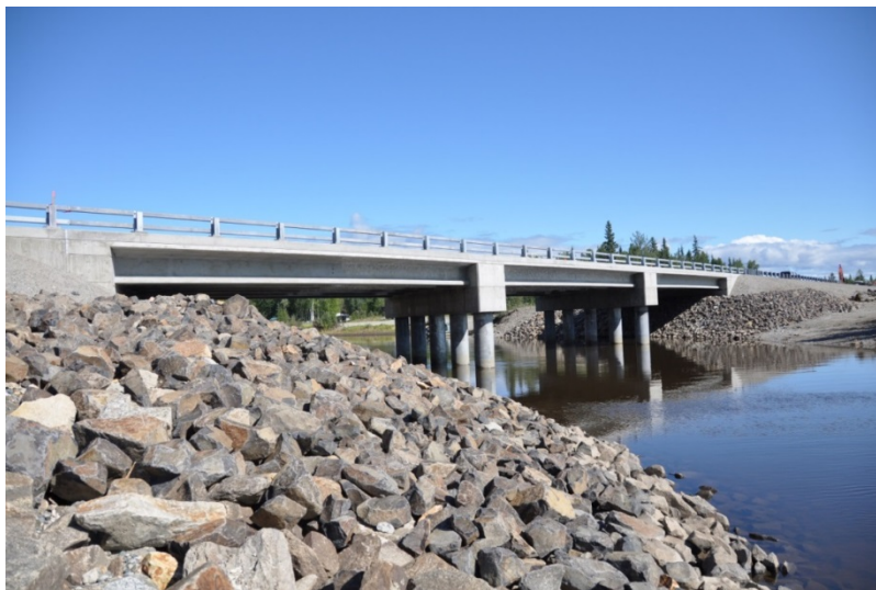
Figure 2 Typical CFST Substructure Units
