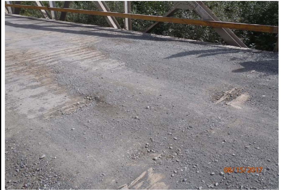
Bridge No. 1193 Br. Name Chokosna River Date 08/15/17 Inspector Levings / Henry Frame 10 NE begin deck with gravel and erosion of wood
