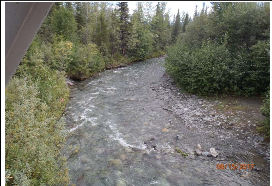
Bridge No. 1193 Br. Name Chokosna River Date 08/15/17 Inspector Levings / Henry Frame 4 Looking DS
