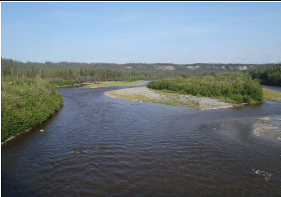
Bridge No. 0574 Br. Name Gulkana River Date 07/14/17 Inspector Murray / Knapp Frame 3 Looking US
