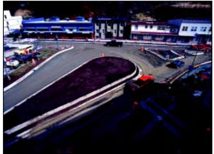
Traffic circle construction, Downtown Juneau, May 2001.
