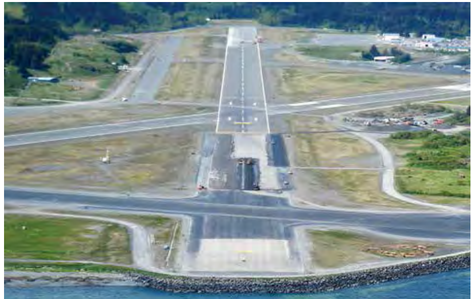
Kodiak Runway 25 under Reconstruction. Photo by Robert Greene ADOT&PF
