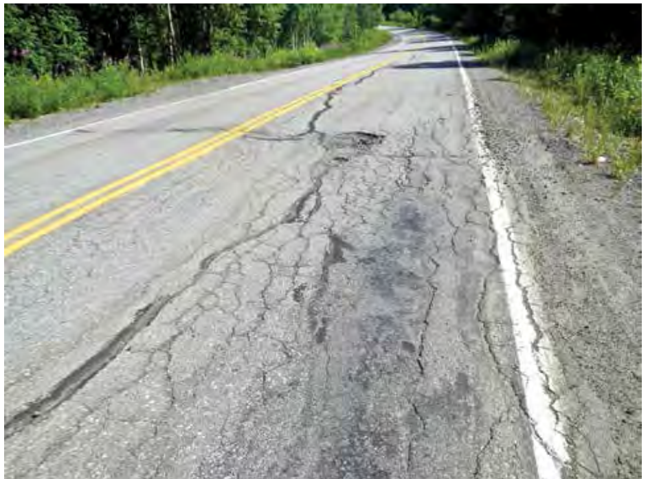
Longitudinal Cracking. Photo by Jim Horn, ADOT&P.
