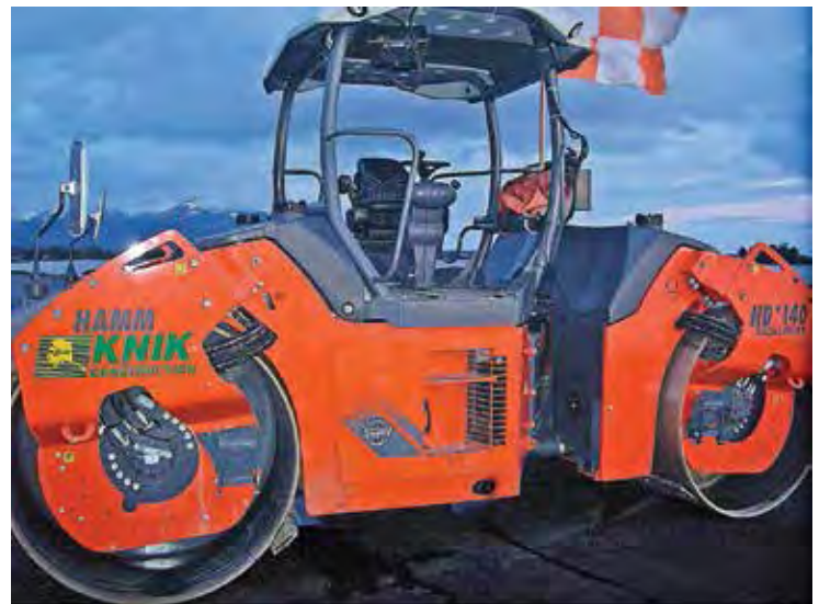
Intelligent compactor rolling asphalt at the Sitka Airport. Photo by Steve Saboundjian, ADOT&PF
