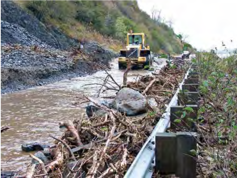
Landslide on Rezanof Drive, Kodiak Photo by Todd Dorman, ADOT&PF
