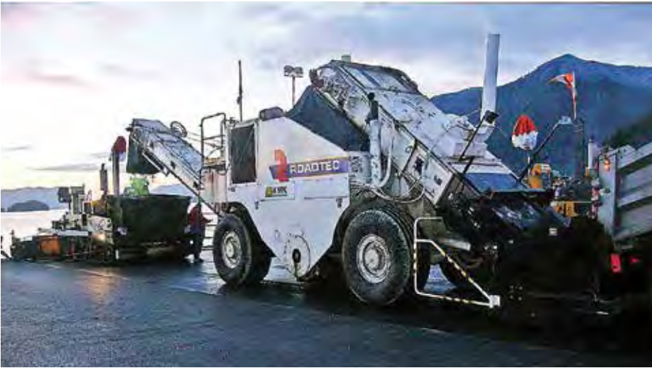
Material transfer vehicle applying asphalt at the Sitka Airport. Photo by Steve Saboundjian, ADOT&PF
