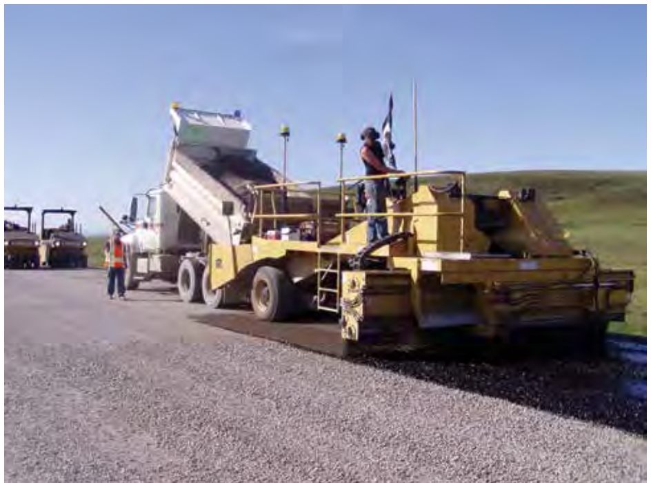
Chip Sealing on the Dalton Highway. Photo by Harold Kremer ADOT&PF
