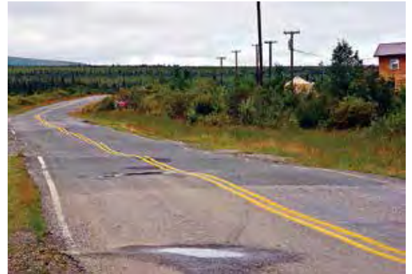
Thawing of permafrost, Stampede Road. ADOT&P archives.
