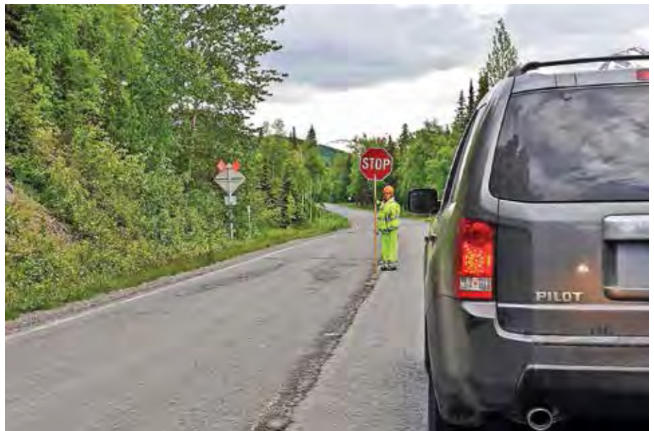
Pavement repair ahead, on the road to Homer. Photo by Kathleen Metcalfe.
