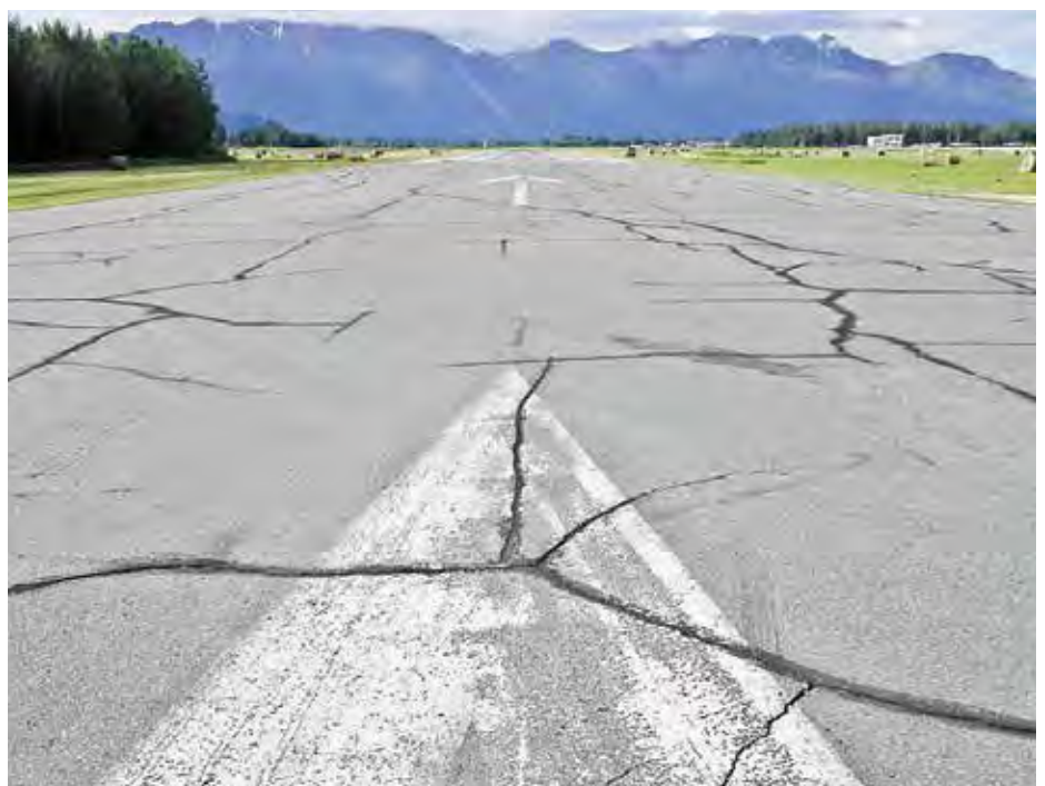
Cracking at the Palmer Airport. Photo by Jim Horn ADOT&PF.
