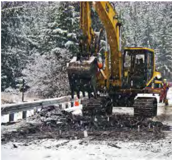
Removing the deck of the Peterson Creek Bridge. Photo by Michael Kell, ADOT&PF.
