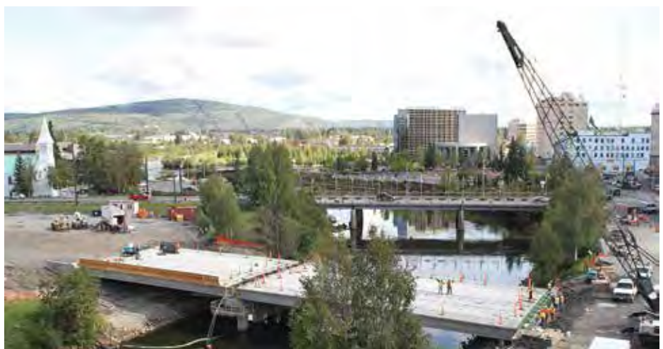
Barnett Street Bridge in Fairbanks. Photo by Meadow Bailey, ADOT&PF.
