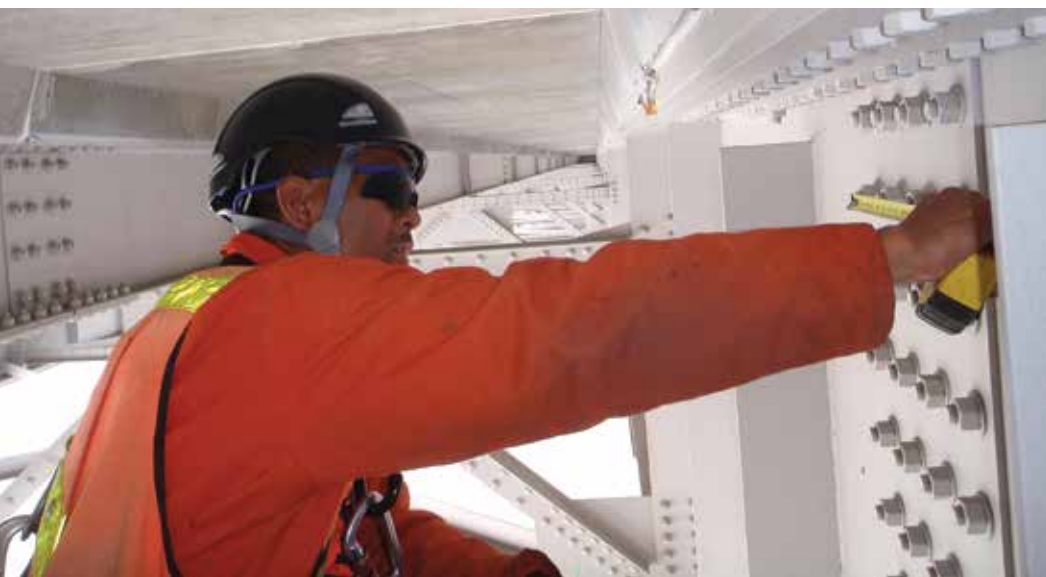
John Orbistondo inspecting the Yuikon River Bridge piers. Photo by Larry Durfee, ADOT&PF.
