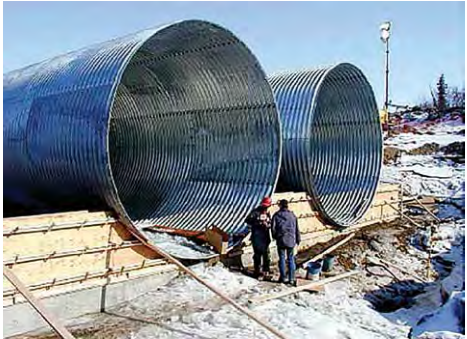
Culverts for the Marshall Airport Access Road. Photo by Clyde Kelso, ADOT&PF.
