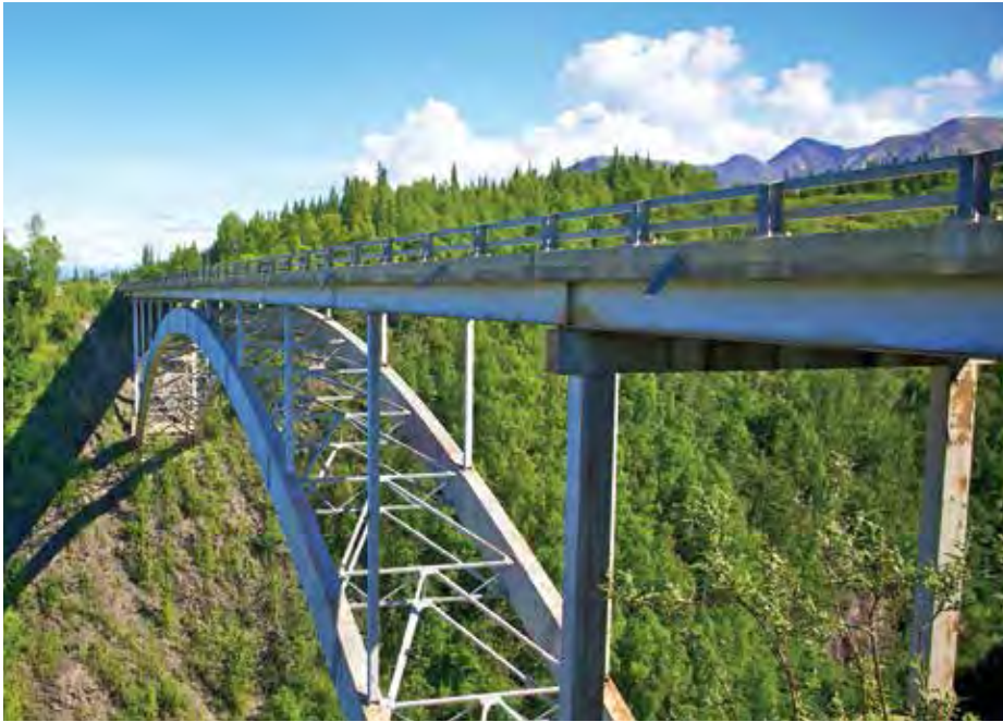
Hurricane Canyon Bridge on the Parks Highway. Scott Sexton ADOT&PF
