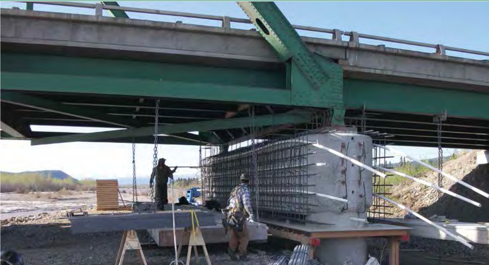
Strengthening a pier on the Nenana River Bridge. Photo by Elmer Marx, ADOT&PF
