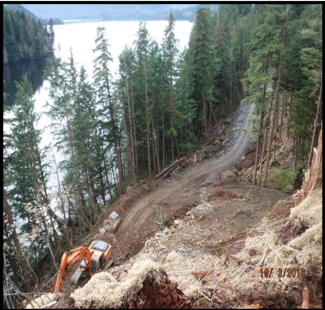
Shelter Cove Road – Pioneer road construction in progress
