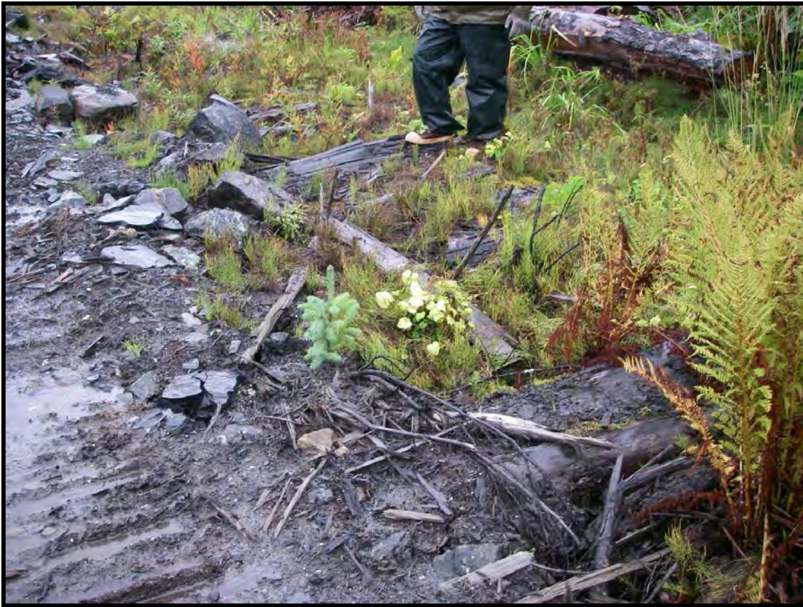
Photo 19: Typical corduroy construction over soft ground.
