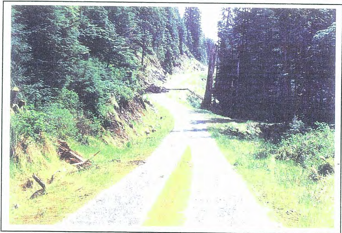
Photo 2 : Typical roadway section showing steep cut slopes in mixed soil and rock common material. Note irregular roadway alignment.
