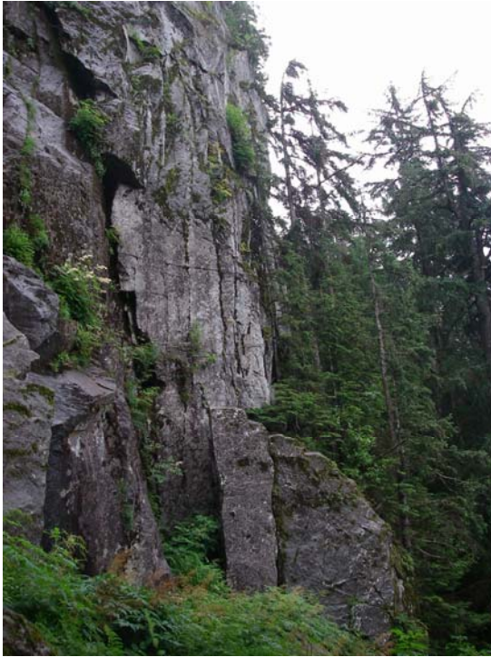
RF33. View south/down alignment at tabular blocks creating rockfall hazard. Photo taken 90 ft right of IRP 2006 2367+00.
