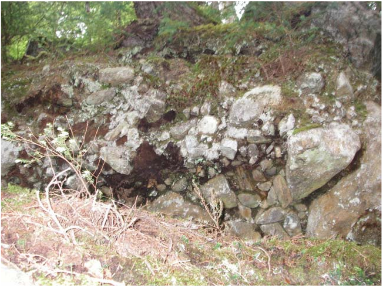
Elevated beach deposits (Qeb) - View upslope at weakly cemented elevated beach deposits. Photo taken at centerline at IRP 2006 2158+00.
