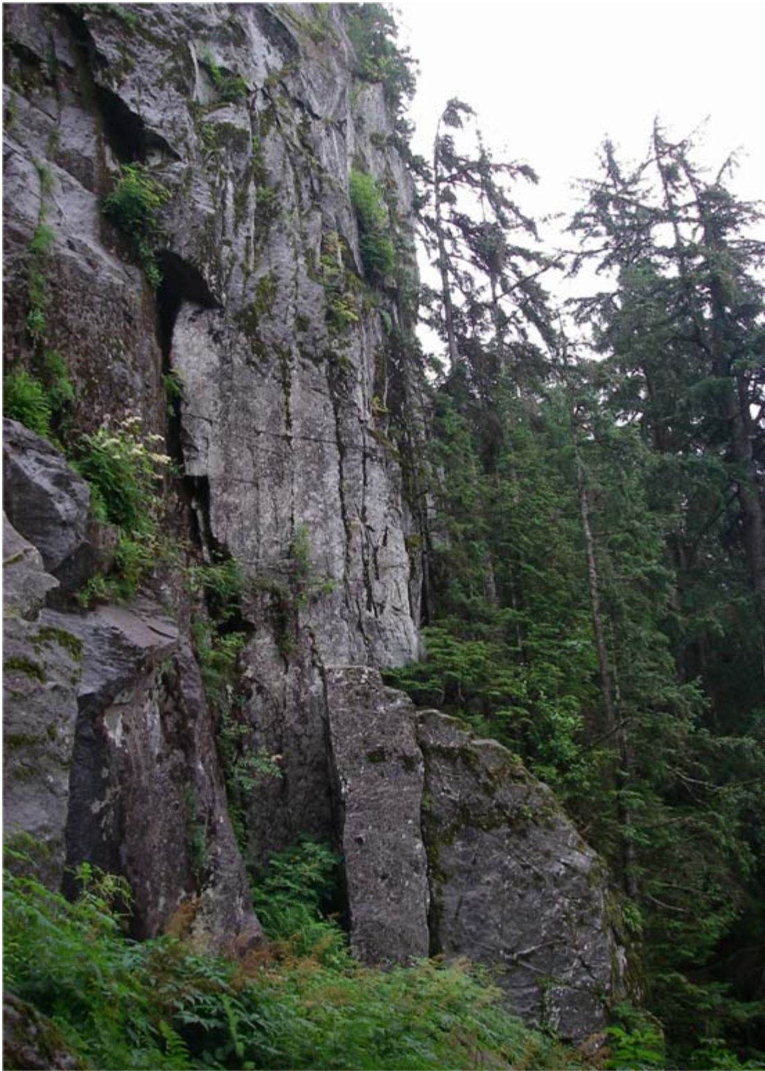
Gneiss bedrock (Bxmg) - View of typical gneiss cliff. Note prominent joint set. Visible cliff is approximately 150 ft tall. Photo taken 100 ft right of IRP 2006 2365+00.
