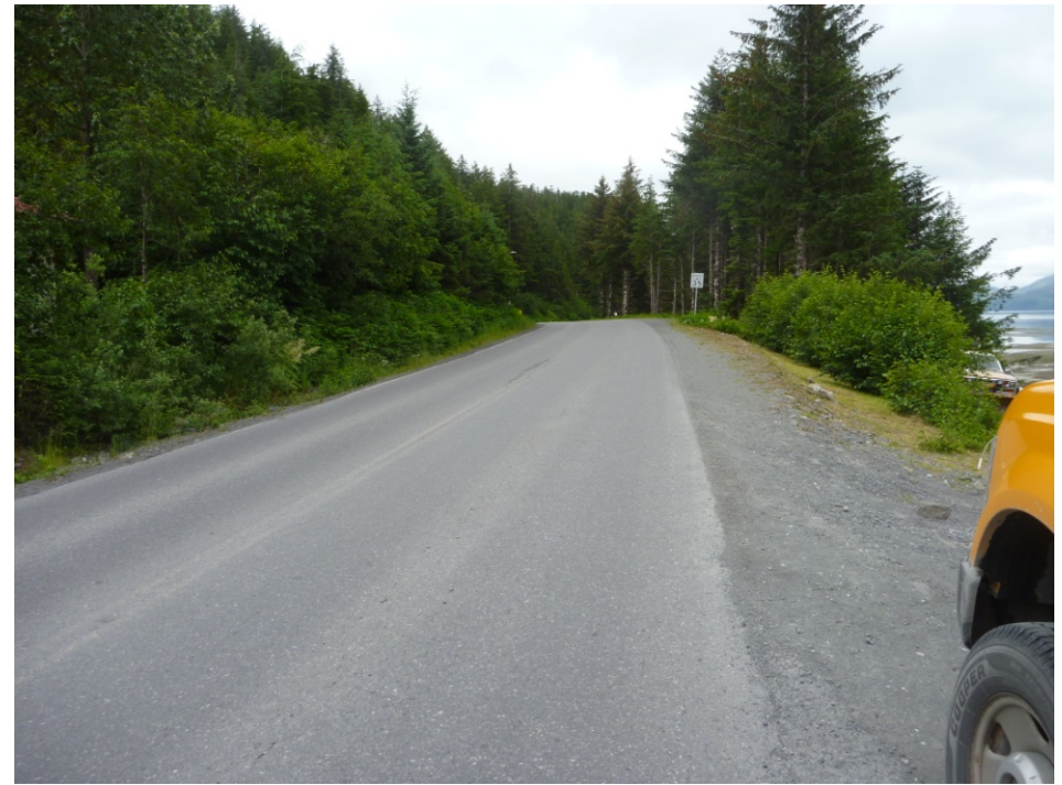
Looking west on Whitshed Road away from Cordova city center. Narrow roadway lanes, no shoulders or pedestrian facilities, steep mountain face on the left, steep drop to the ocean on the right.
