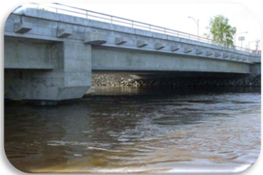
Barnette Street Bridge, July 2011
