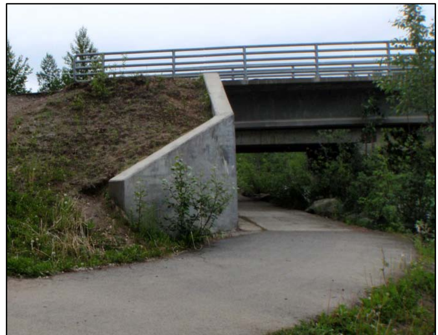
Vertical Wall Abutment
