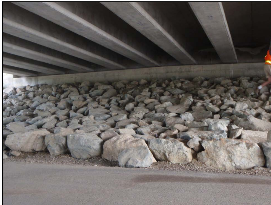
“Spill Through” Sloped Abutment
