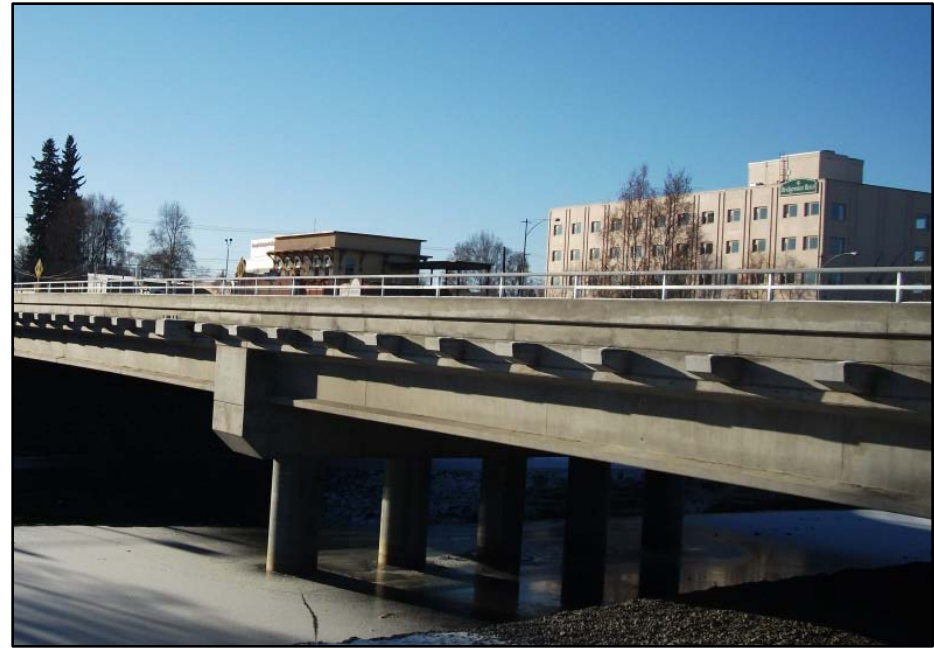
Barnette Street Bridge
