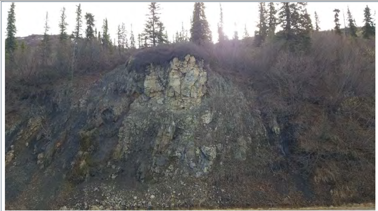
Photo 5: MP 212.3 Potential rockfall hazard.
