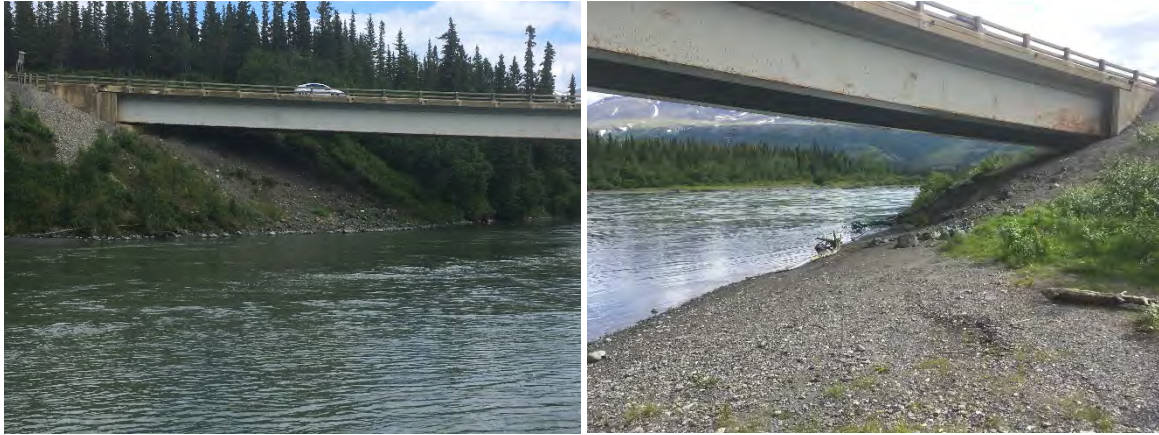
Figure 7. Looking Upstream, Left and Right Abutment
