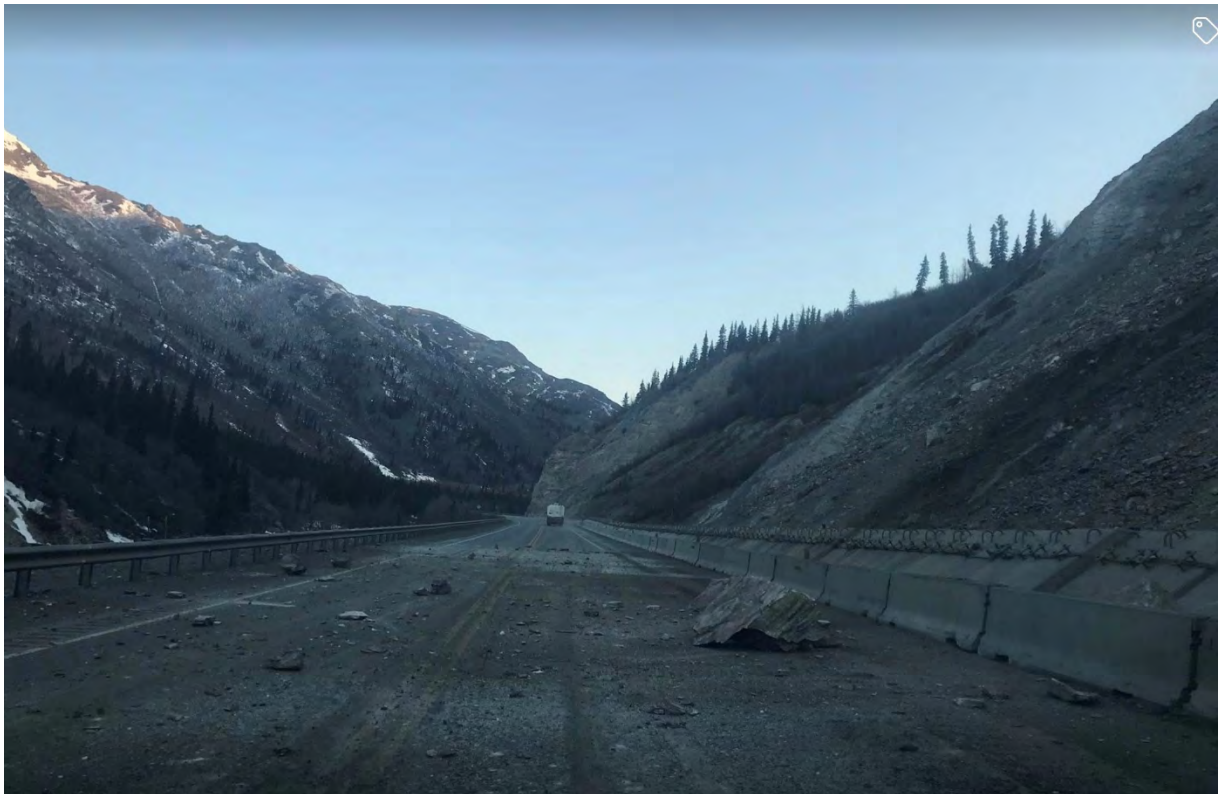
Figure 17 – Larger rockslide that has traveled onto the Parks Highway in Nenana Canyon
