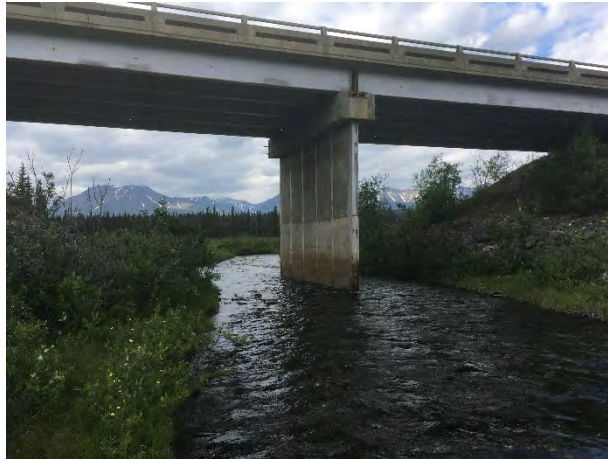
Figure 2. Pass Creek Bridge (BR 0293) Upstream Looking Downstream
