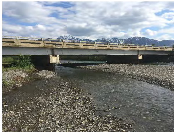
Figure 4. Jack River Bridge (BR 0293) Downstream Looking Upstream
