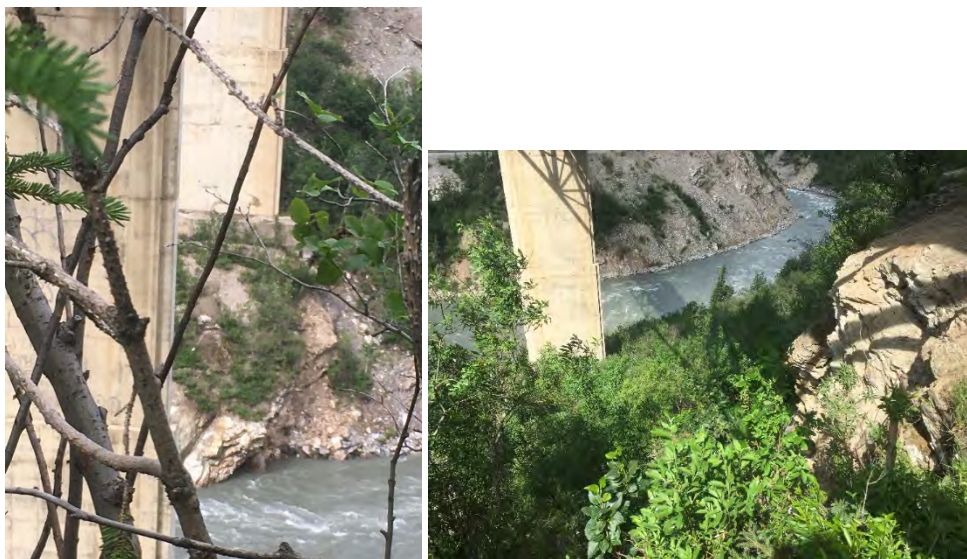
Figure 34. Looking Downstream, Left Pier and Right Abutment
