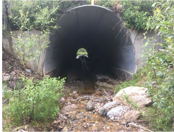
Figure 28. Eagle Creek Cross Culvert (7111/1076), Upstream Looking Downstream
