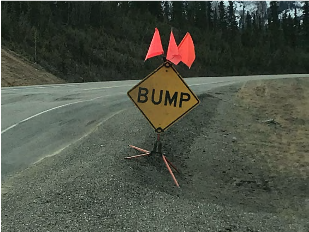
Figure 7 - Additional photo of bumpy section near MP 232.5
