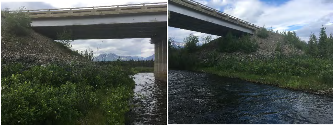
Figure 3. Looking Upstream, Left and Right Abutments
