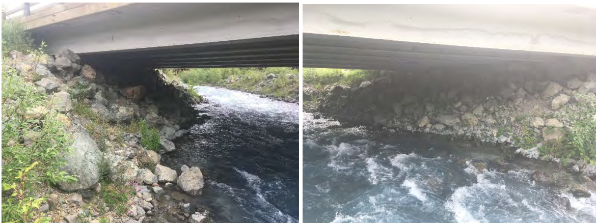
Figure 11. Looking Upstream, Left and Right Abutment
