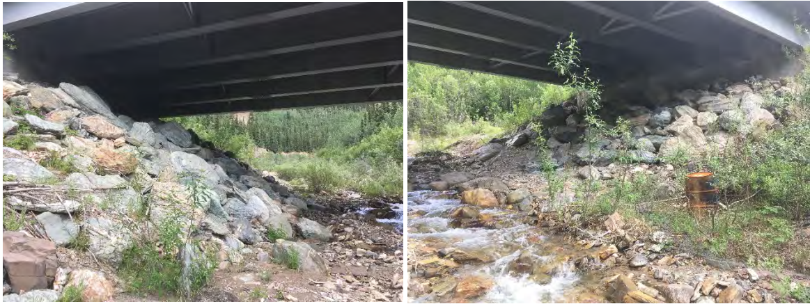
Figure 24. Looking Upstream, Left Abutment and Right Abutment
