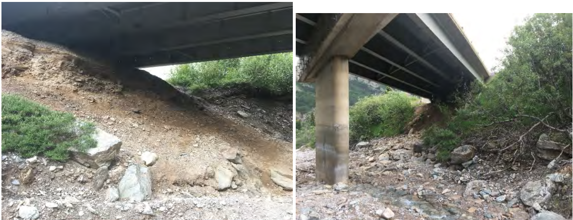
Figure 36. Looking Downstream, Left and Right Abutment
