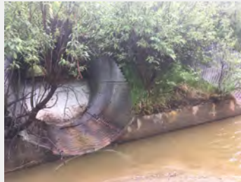
Culverts at Slate Creek (MP257.8), shown here, and Little Panguingue Creek (MP 254) are identified by ADF&G as poor for overall fish passage
