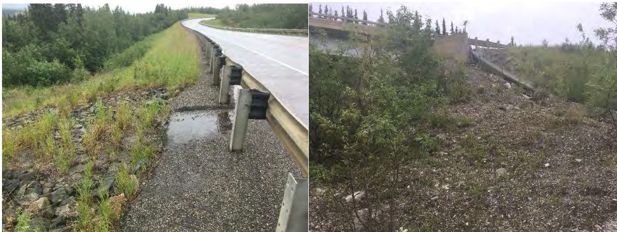
Figure 62. Typical Riprap Flume Looking Toward Slate Creek: Typical Metal Flume on Southbound Side of the Kingfisher Creek Crossing
