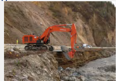
Rockfall, drainage, and sediment build up are continuous issues along the highway in Nenana Canyon (MP 239-240)
