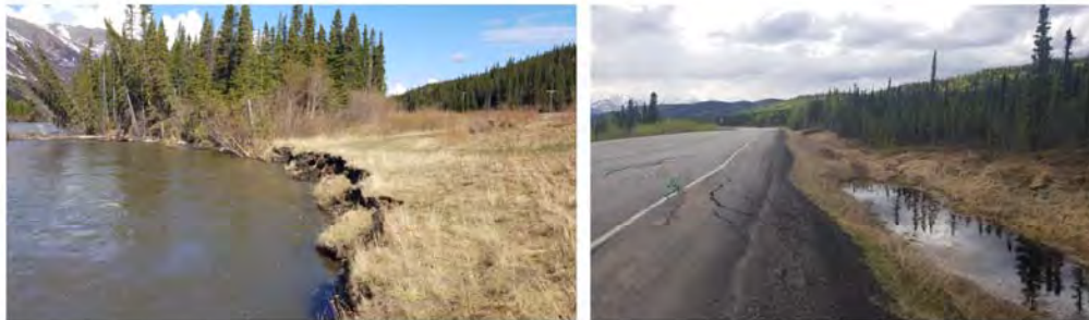
Bank erosion from Nenana River adjacent to the Highway (MP 222.8) (Left), Roadway deterioration adjacent to thaw pond, likely caused by thawing permafrost (MP 256.4) (Right)
