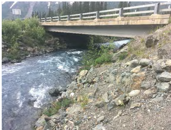
Figure 10. Carlo Creek Bridge (BR 0693), Upstream Looking Downstream
