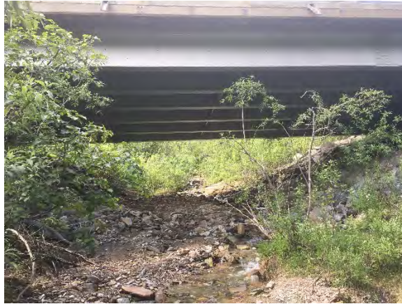
Figure 30. Dragonfly Creek Bridge (BR 1075), Downstream Looking Upstream
