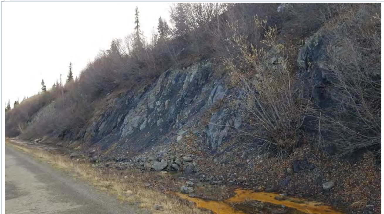
Photo 6: MP 212 Unstable soil and rock slope. Vern Carlson (Maintenance Foreman) stated that the site was a slow-moving slide that caused the ditch to be cleaned out every three to five years depending on rainfall.
