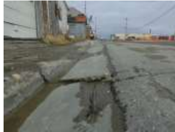
Cracking pavement in Nome, AK
