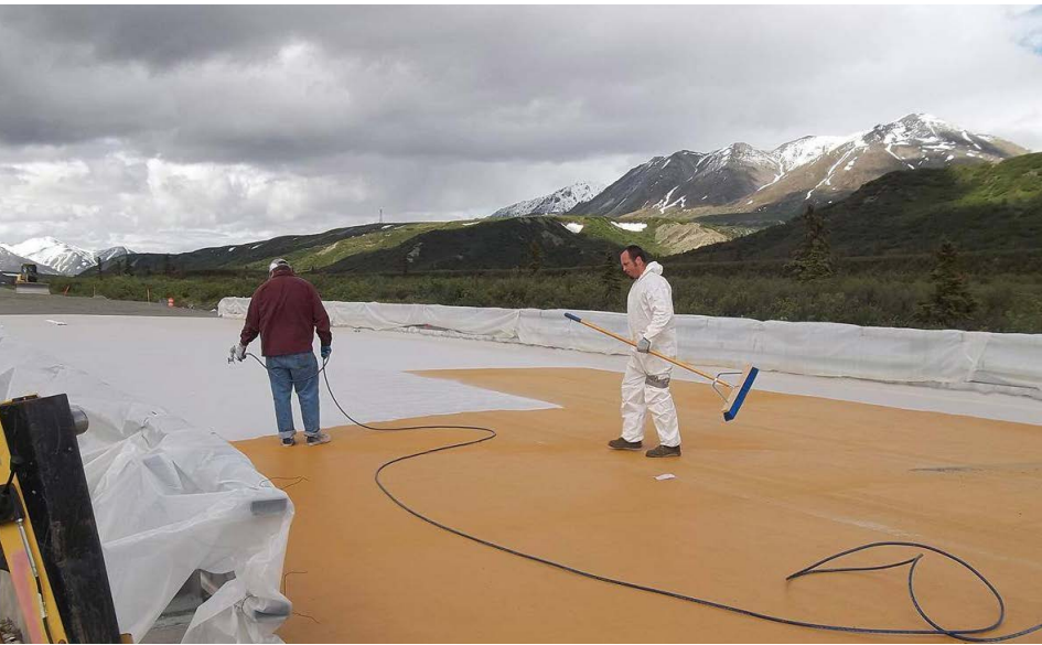
The second (gray) layer of membrane is applied on top of the first (yellow) layer. Photo by Raquel Ream, DOT&PF
