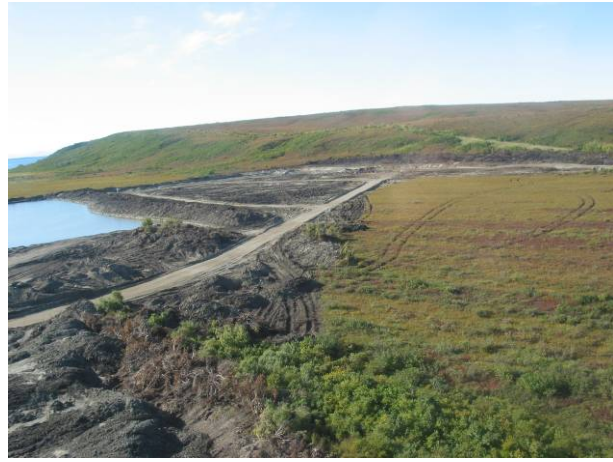
Figure 10 Material site development. Access road to oil exploration pad in background
