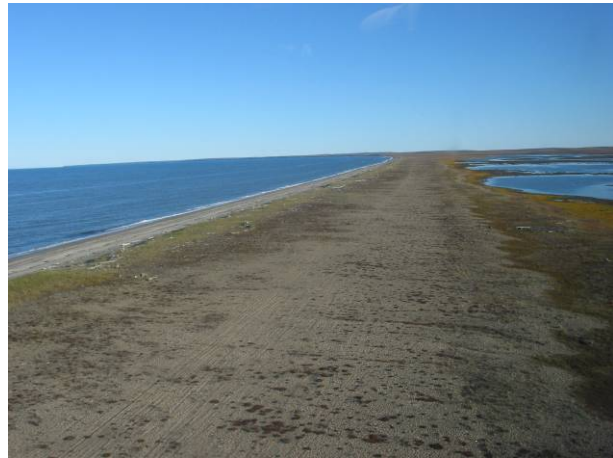
Figure 12 Arctic Circle Strip (Jeppsons Strip), 12,000 feet of straight wide gravel, 4800 feet between threshold markers
