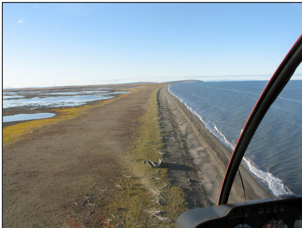
FIGURE 15: ARCTIC LANDING STRIP (View South; 31 August 2006)
