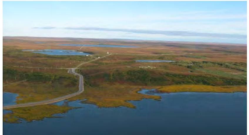
Photo 2-2 Ted Stevens Way, Vortac Road, and Hillside Road
