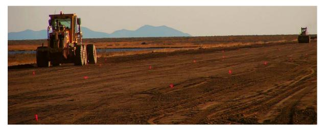
FIGURE 10 - CONSTRUCTION OF A SILT EMBANKMENT AT ALAKANUK AIRPORT (SEPT. 2008)
