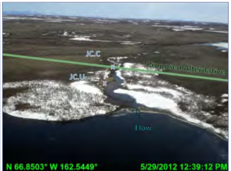
PHOTO 4.17: DISMISSED UNNAMED SWALE CROSSING, LOOKING NORTHEAST; MAY 29, 2012
