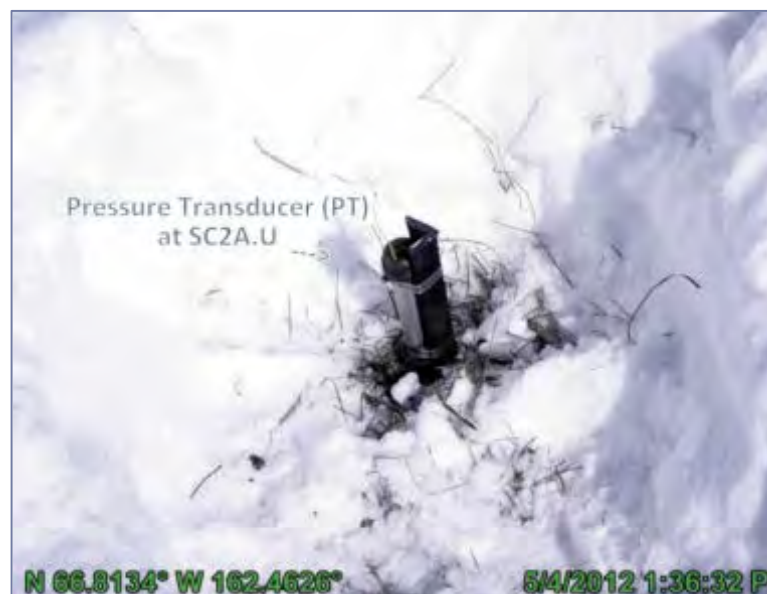
PHOTO 3.2: PT ASSEMBLY INSTALLED AT SC2A.U; MAY 4, 2012
