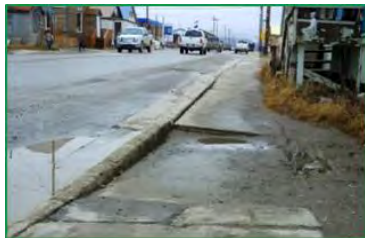
Example of road shoulder and sidewalk deterioration.
