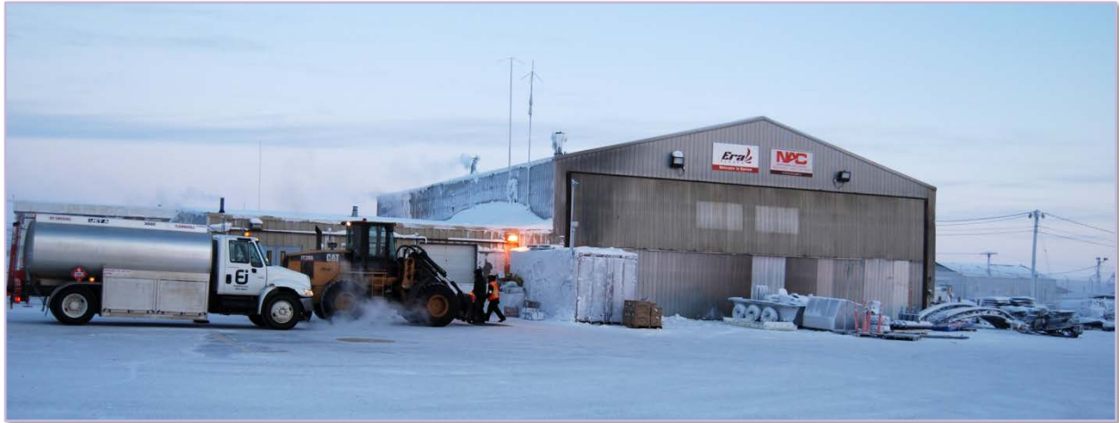
Figure 2-9 – Era Aviation Cargo Handling Facility at BRW
