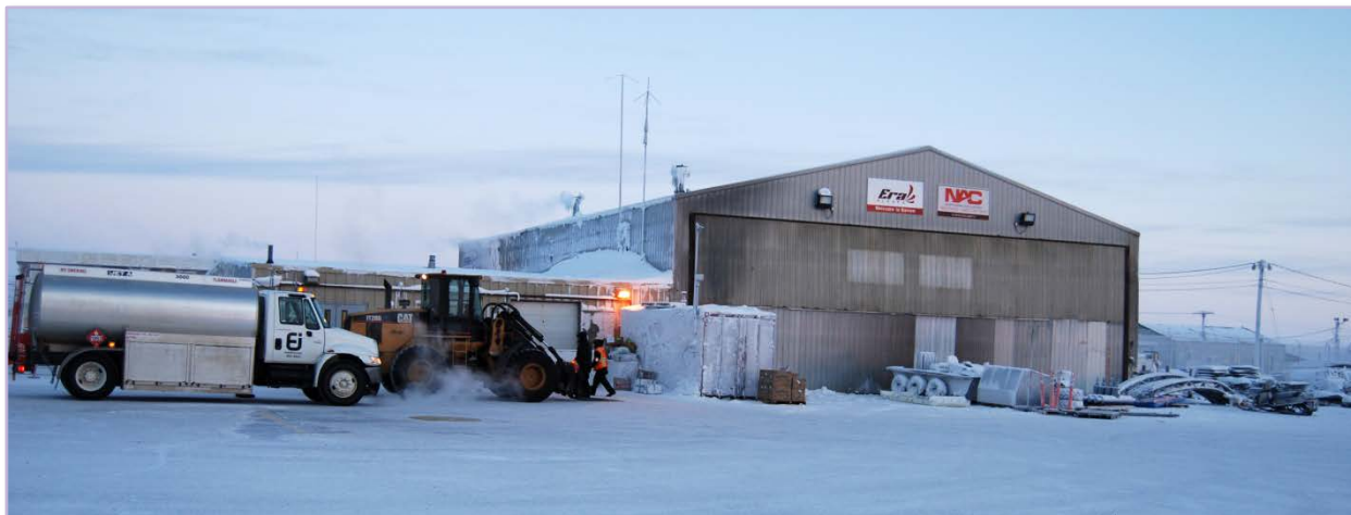
Figure 2-9 – Era Aviation Cargo Handling Facility at BRW
