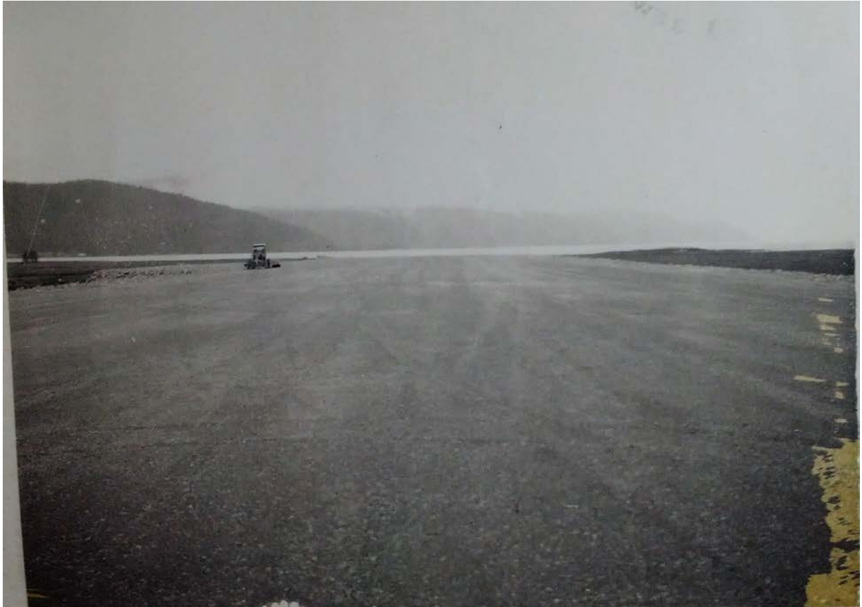
Figure 11. Overview of southern end of runway 13-31 after DOT&PF had 75% compaction from contractor in July 1966, facing southeast. Photo from DOT&PF archives.
