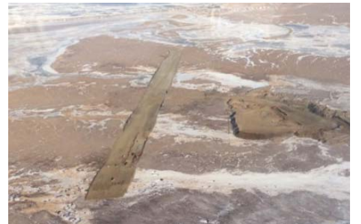
New Tununak Airport embankment
