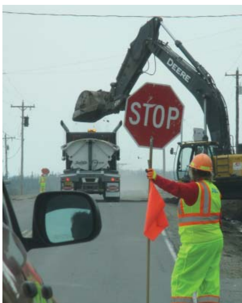
Work site construction
