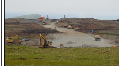
Akun Island Airport construction Summer 2011
