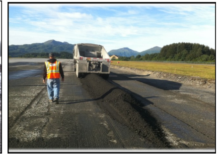
Kodiak Airport Construction placing Foamed Recycled Asphalt Pavement
