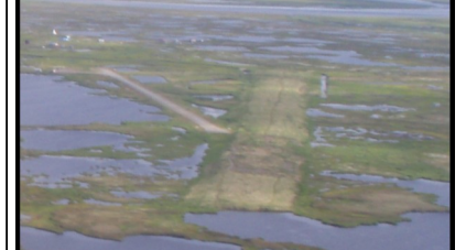
Kipnuk Airport Embankment Summer 2009
