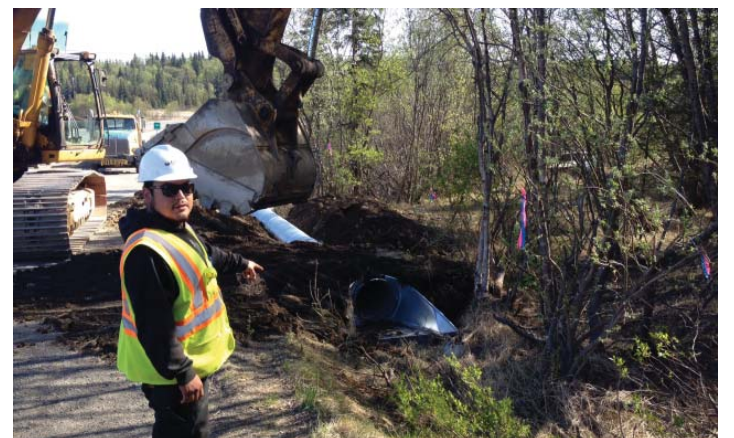
Culvert replacement at the "Y" off Kanakanak Road
