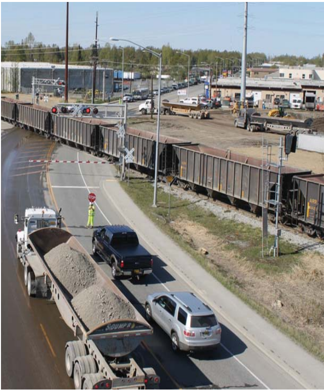
Keeping traffic moving during construction of the West Dowling Road Extension project is more challenging due to the need to accommodate rail traffic. Also, note the extensive utilities that needed to be accommodated and addressed in the design.
