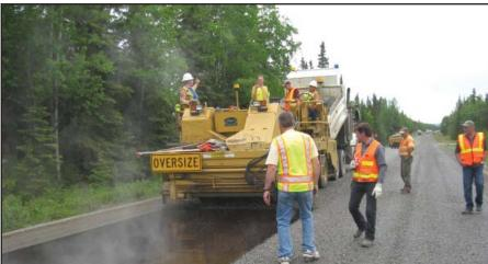
ADOT&PF applying test section of Cohoe Loop Road in Kasilof this June. Chip-seal resurfaces the roadway without the use of asphalt and is meant to last for 10 years of wear.
