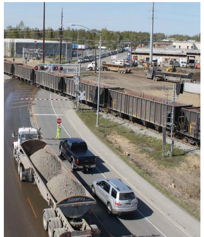
Keeping traffic moving during construction of the West Dowling Road Extension project is more challenging due to the need to accommodate rail traffic. Also, note the extensive utilities that needed to be accommodated and addressed in the design.
