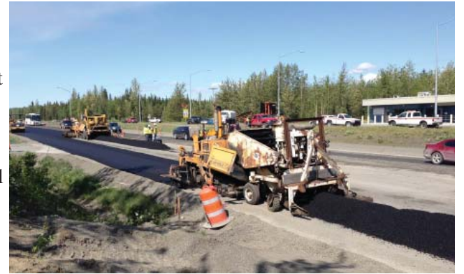
Sterling MP 79-82 Pavement Represervation Project
