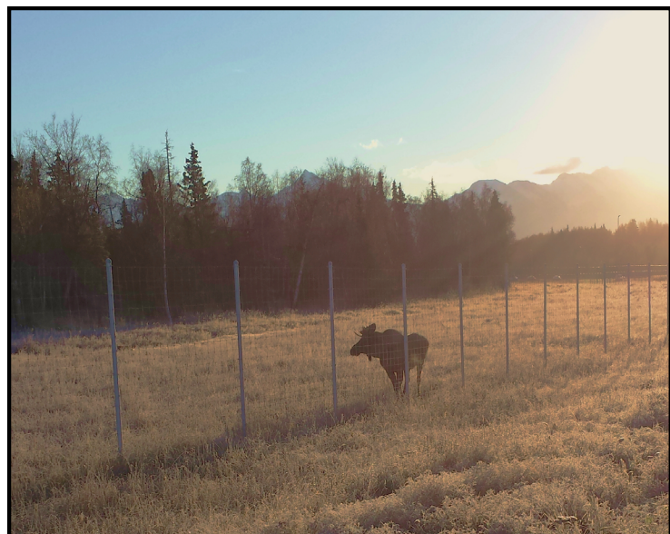
A moose separated from the highway by the newly installed moose-fencing along Minnesota Drive in Anchorage.
