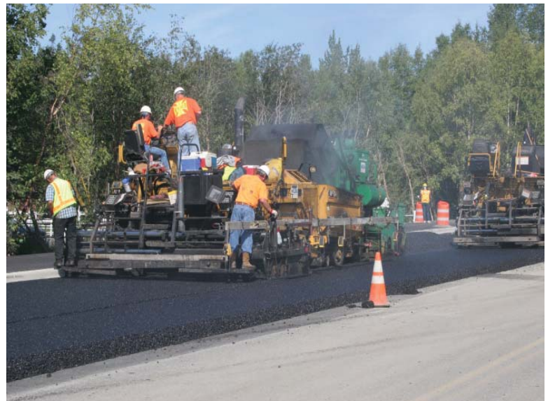
Experimenting with pavement design has led to unanticipated benefits. The rubberized asphalt used on Elmore Road (shown here being laid in 2007) shed ice much more rapidly than other pavements.
