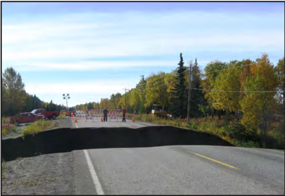
Kalifornsky Beach Road on the Kenai Peninsula required $1.5 million to replace the washed-out road and culvert at MP 11. This segment of road was reopened to traffic 5 days later.
