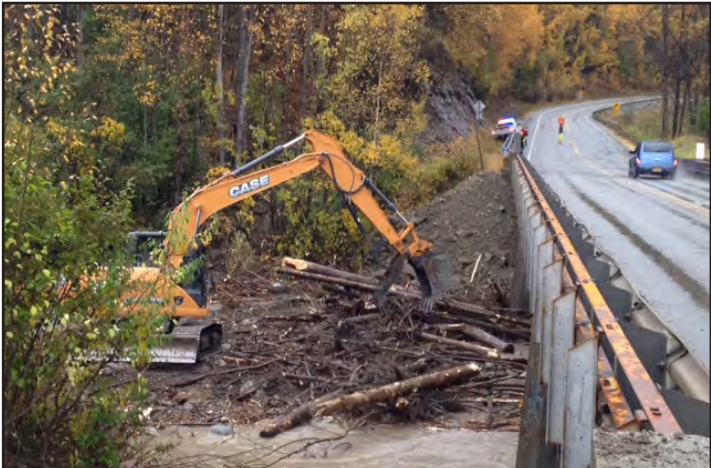
DOT&PF crews clear debris from Moose Creek Bridge on the Glenn Highway north of Palmer during the flood to prevent a washout of the bridge.
