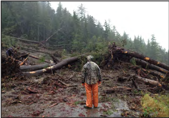
Fallen timber and a mudslide 70 feet wide block Chenega Bay's access to its airport. The local DOT&PF contractor spent almost a week reestablishing the road connection for this Prince William Sound community.
