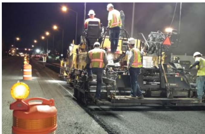
Downtown pavement replacement work was accomplished at night to minimize travel disruptions.
