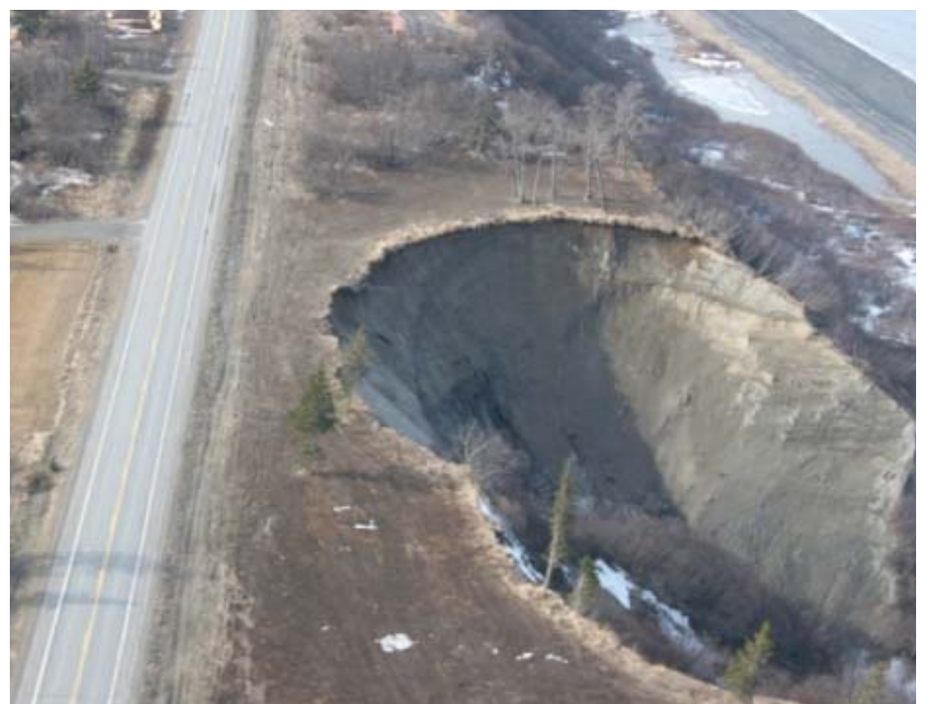
The Department is currently requesting bids to address the erosion at MP 153 of the Sterling Highway.
