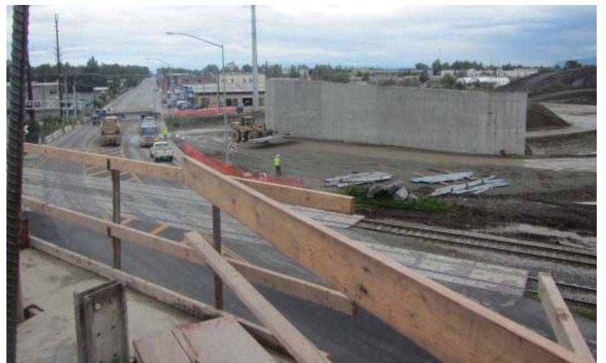
Bridge abutments nearing completion. Bridge structure will cross over Arctic Boulevard and the Alaska Railroad lines.
