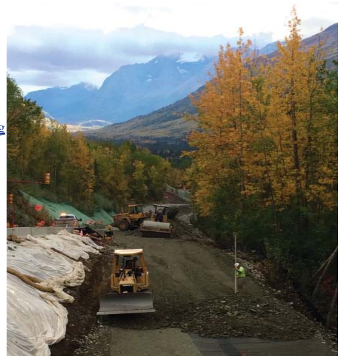
Building up the road bed at MP 6.7 of Eagle River Road as fall colors emerge.
