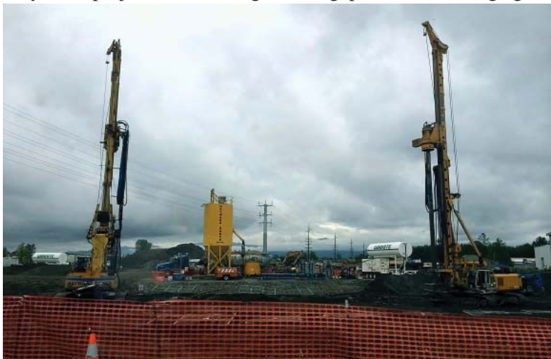
Construction work to stabilize the sub-grade for bridge abutments on the West Dowling Road Phase II project
