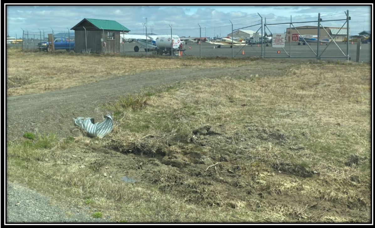
Figure 34: Culvert by GA Apron Access Point
