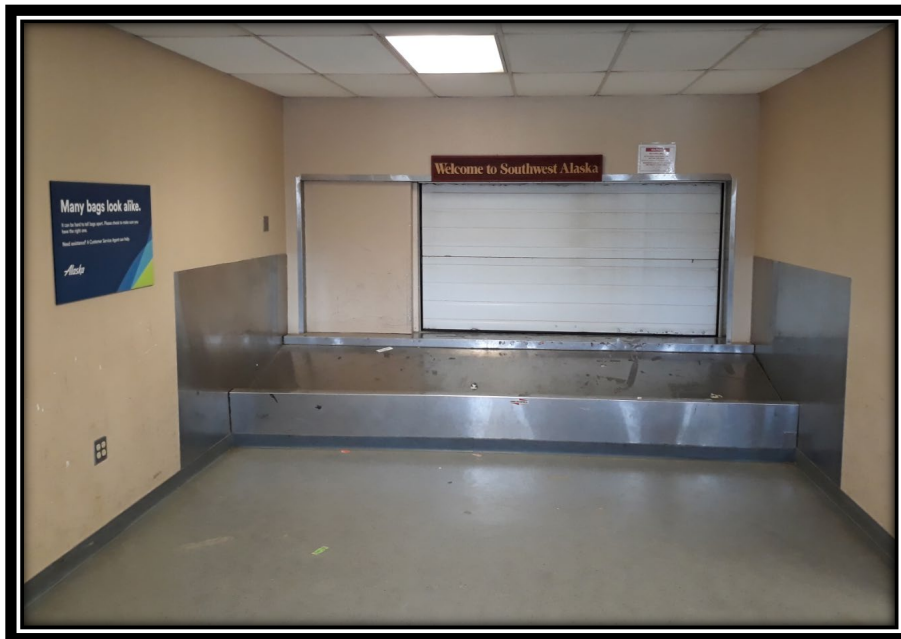
Figure 7: Baggage Claim Area, Alaska Airlines/Ravn Air Terminal Building
