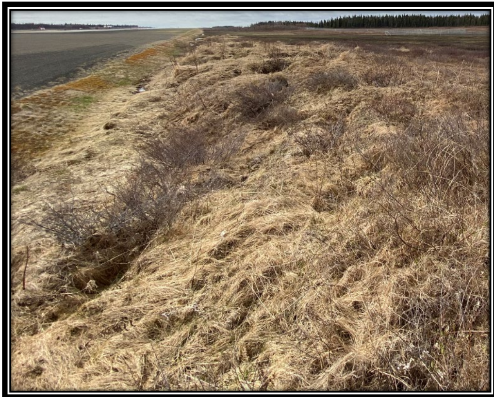
Figure 35: Surface Irregularities in the Tundra Surrounding the Airport Embankment
