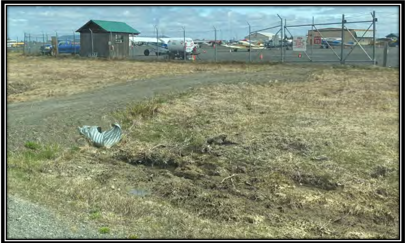
Figure 19: Culvert by GA Apron Access Point
