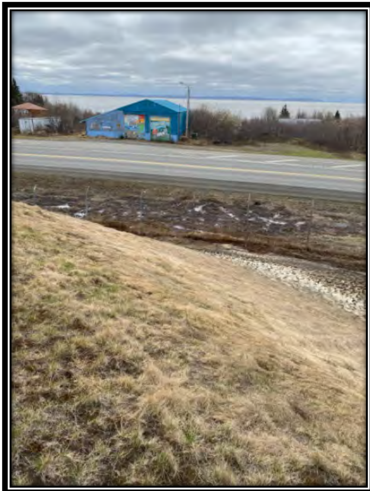
Figure 17: RSA Embankment Slope, RW 1 End Looking Southeast
