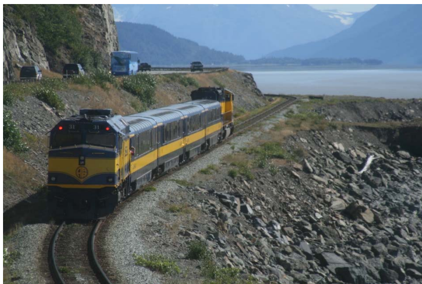
Photograph 3: Alaska Railroad track along Turnagain Arm
