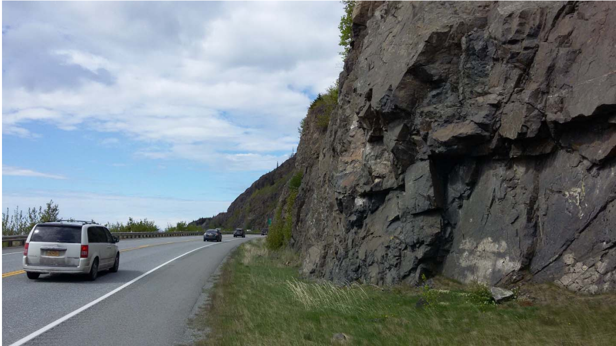
Photograph 10: Former Construction Cut Faces on Seward Highway, MP 111
