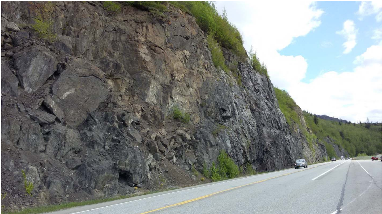
Photograph 9: Former Construction Cut Face on Seward Highway, MP 113
