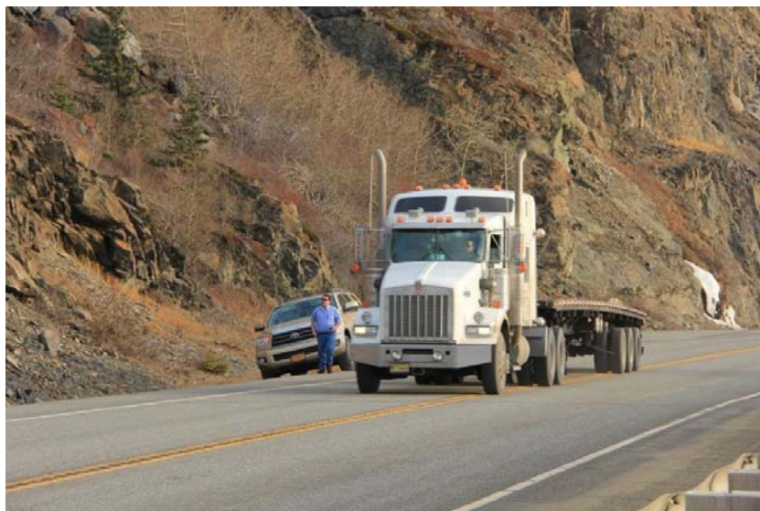
Photograph 8: Seward Highway, Windy Corner Wildlife-Traffic Issues
