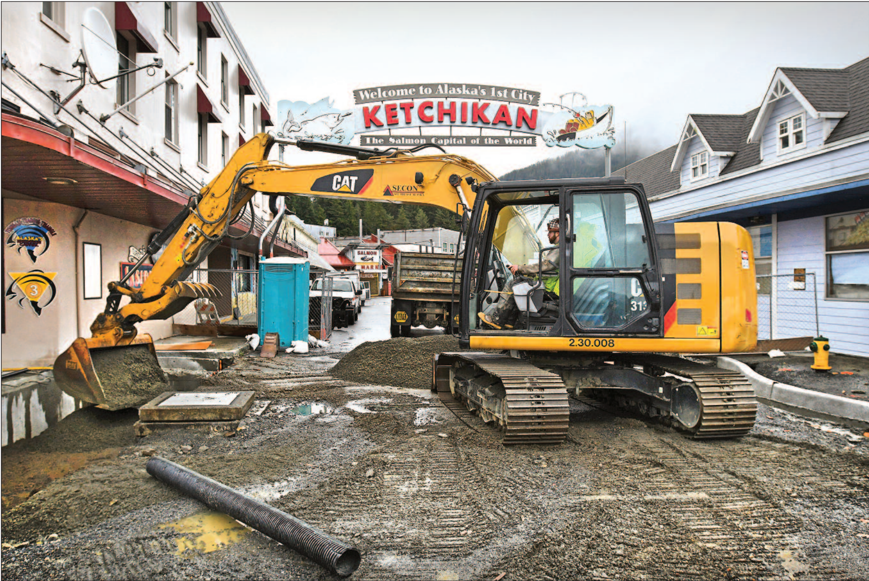
SECON crew member Stewart Meeks uses an excavator to back fill and make sidewalk grade on Tuesday at the intersection of Front and Mission streets.
