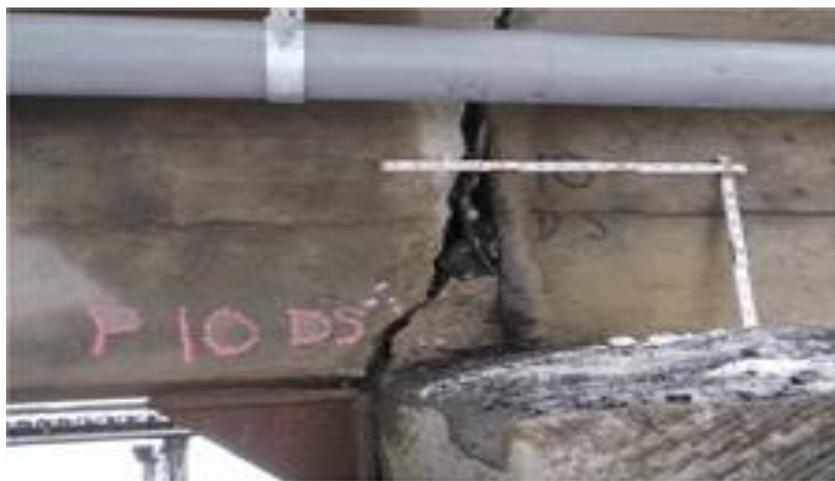
Figure 6. Deteriorating Concrete Trail River Bridge
