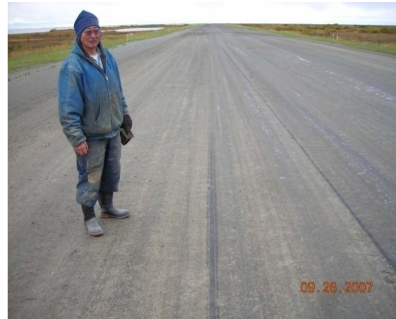
After Dust Control. Our Airport M&O contractor, after chemical dust palliative application. Happy with his runway skid marks!
