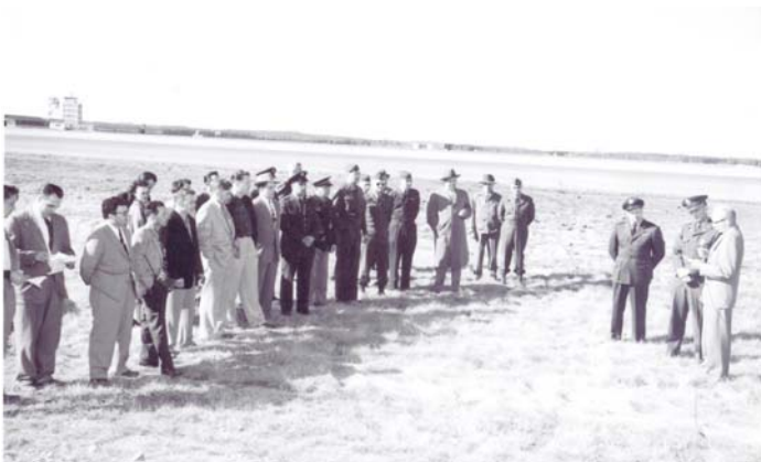
Above: Civilian and military officials gather at Anchorage International Airport to witness groundbreaking ceremonies at the site of the new $717,746 Alaska Air National Guard Hanger and Facilities
